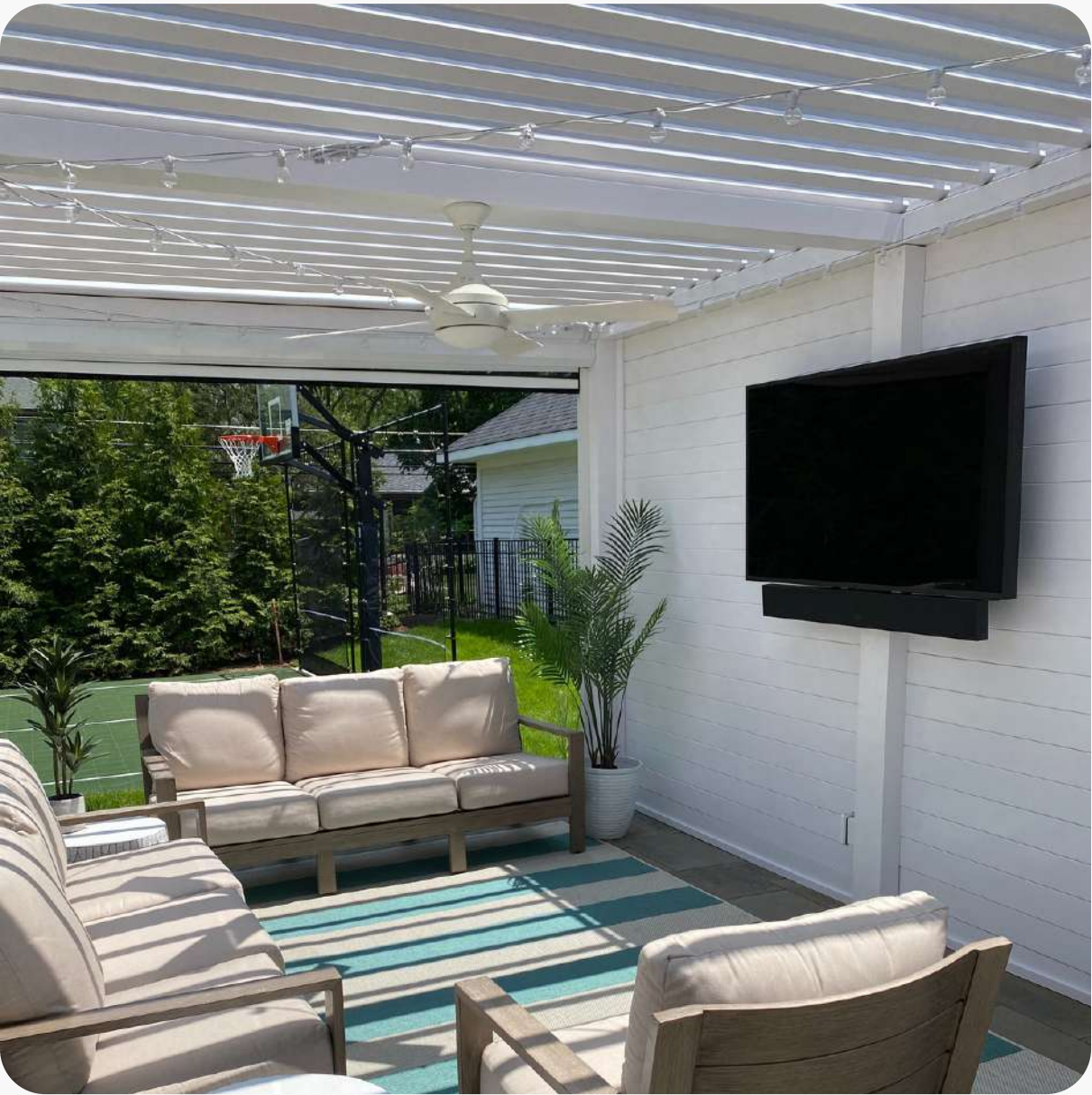
CENTER BEAM For any dimension over 10', a center beam is required to avoid sagging.
